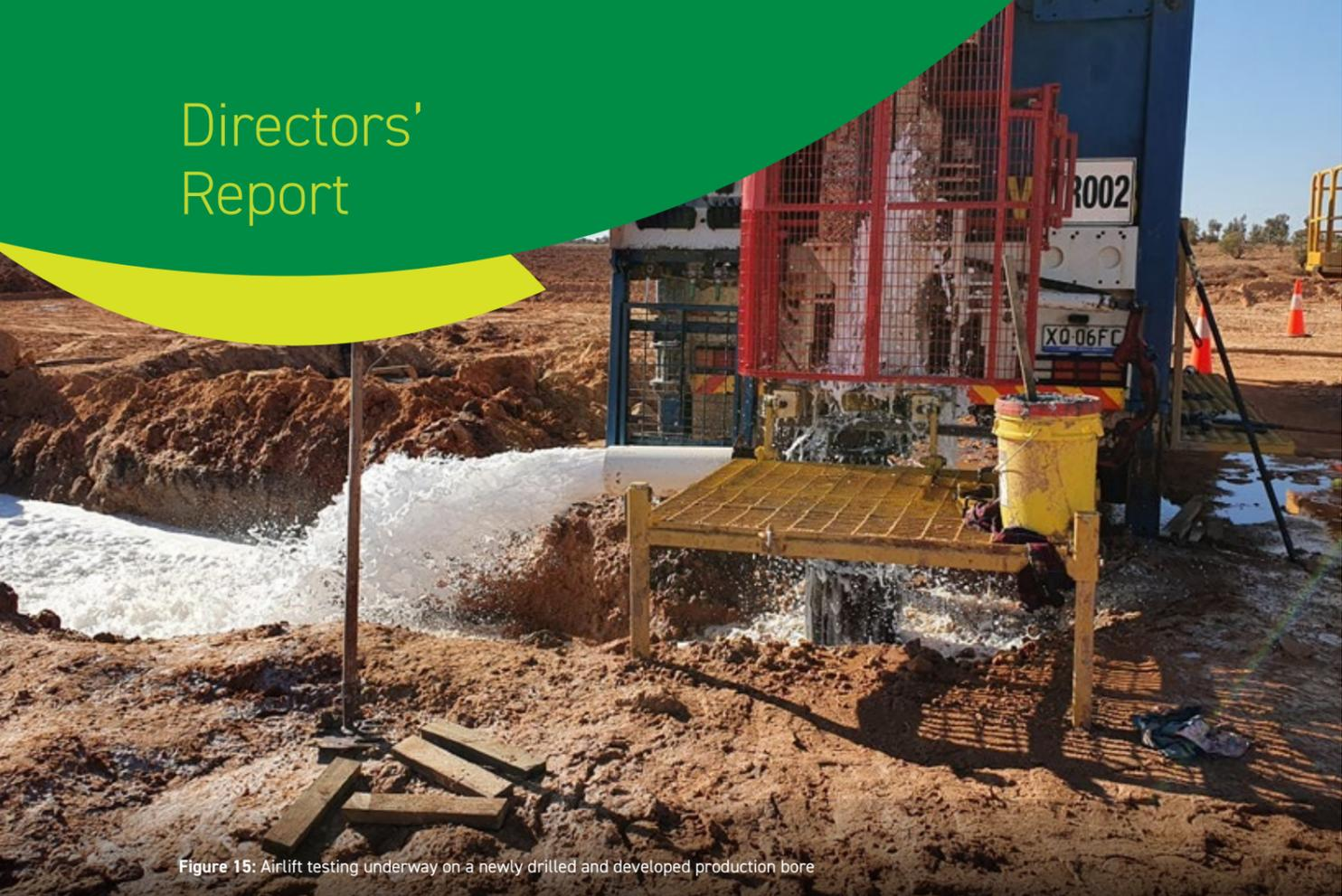
Figure 15: Airlift testing underway on a newly drilled and developed production bore
