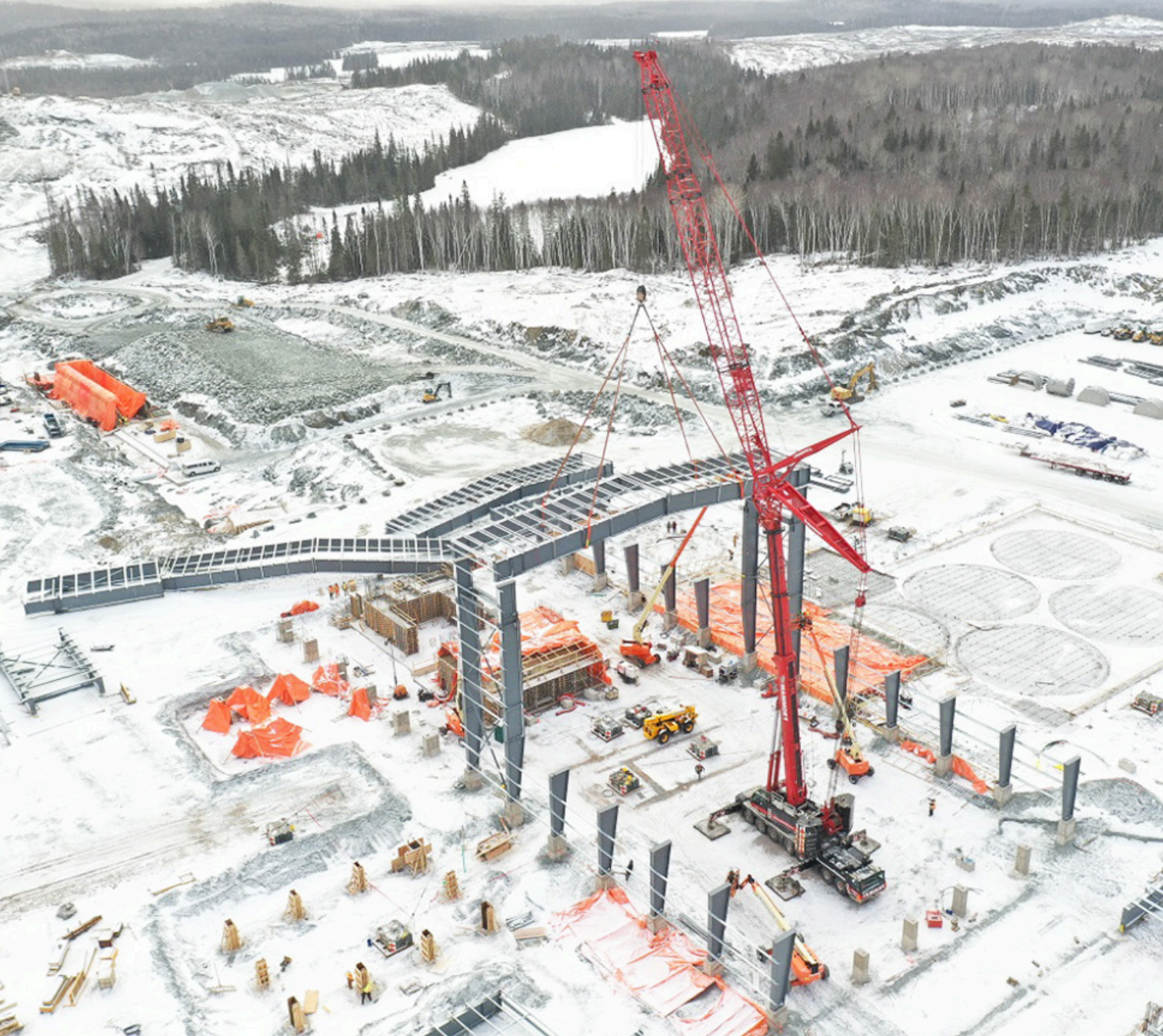
First steel lift at Magino in early 2022.
