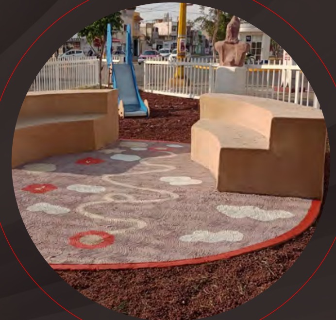
Rehabilitation of a community park in Neza, Mexico.
