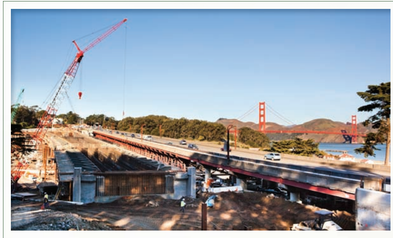
→ DOYLE DRIVE CONSTRUCTION, SAN FRANCISCO, CALIFORNIA ←
