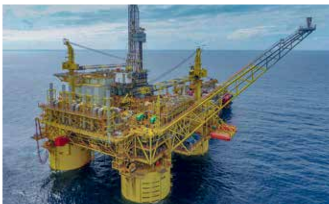
Malikai deep-water platform, Malaysia.
