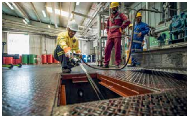
Shell lubricant plant, Oman.
