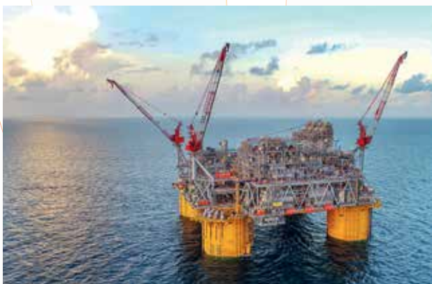
Production has started at Shell's Appomattox deep-water asset in the US Gulf of Mexico.
