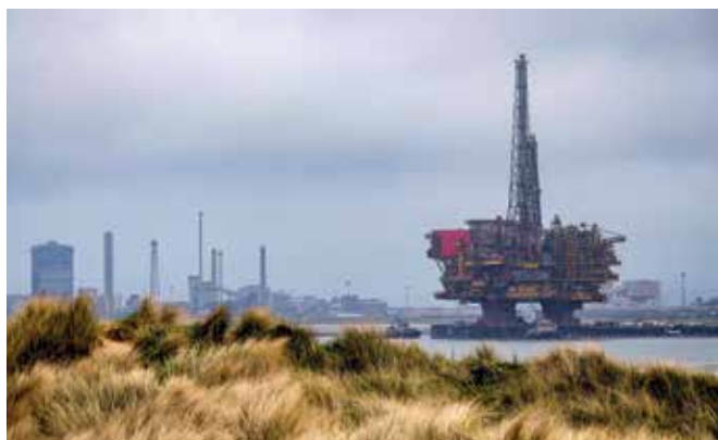
Brent decommissioning using Allseas Pioneering Spirit, the world's largest construction vessel.
