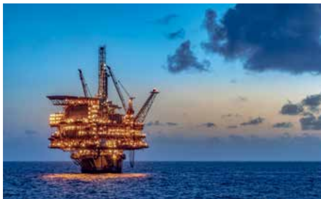
Perdido offshore deep-water platform in the Gulf of Mexico.
