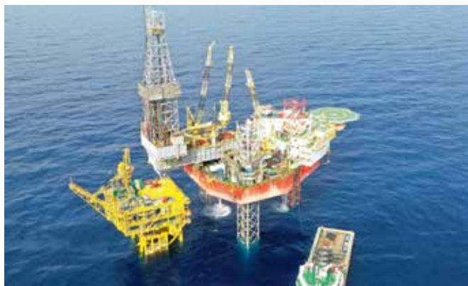
First oil and gas for phase 2 of the E6 project in Malaysia is expected in 2021.
