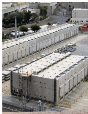
Photos, from left to right: ■ Edison Energy helps companies limit risk from energy price fluctuations with wind and solar contracts. ■ After a period of review, SCE restarted the transfer of spent fuel to dry storage at San Onofre Nuclear Generating Station, which was retired in 2013.
