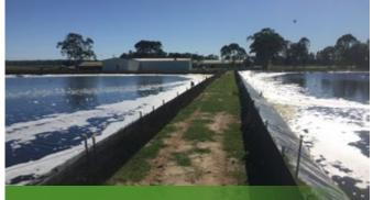
Prawn ponds at Yamba, NSW have been excavated, fully lined, irrigated, fenced and filled from the nearby Clarence river.
