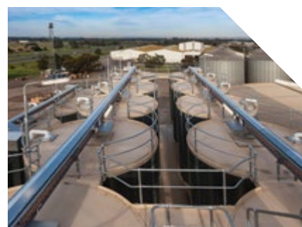
Lara feedmill storage silos.
