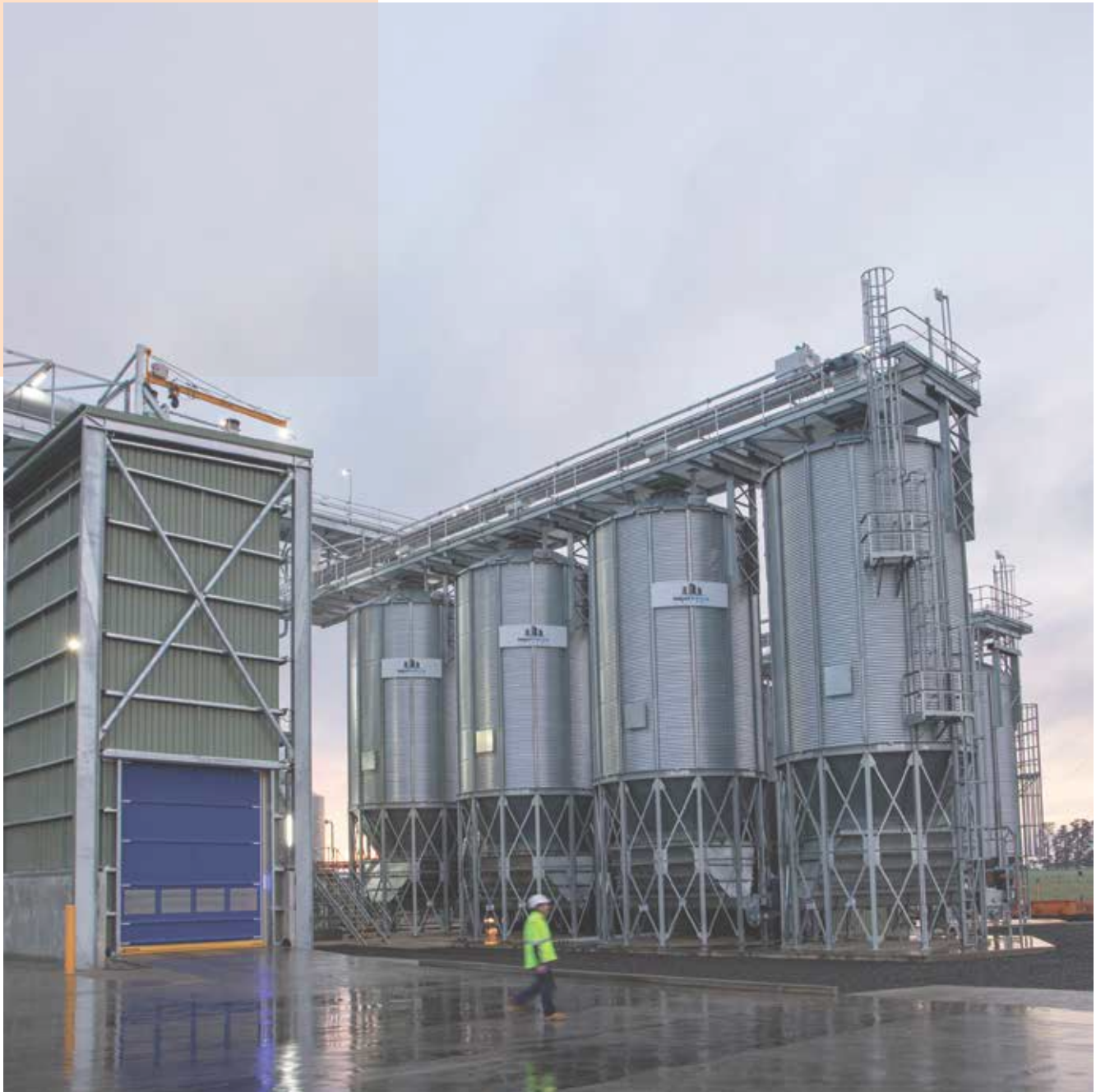
New extrusion plant at Westbury, Tasmania
