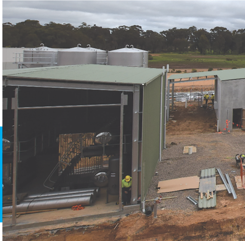
August 2019 progress at the Wellsford site, Bendigo, Victoria
