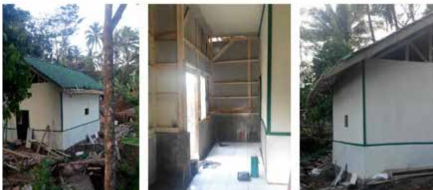
Veteran house renovation.
