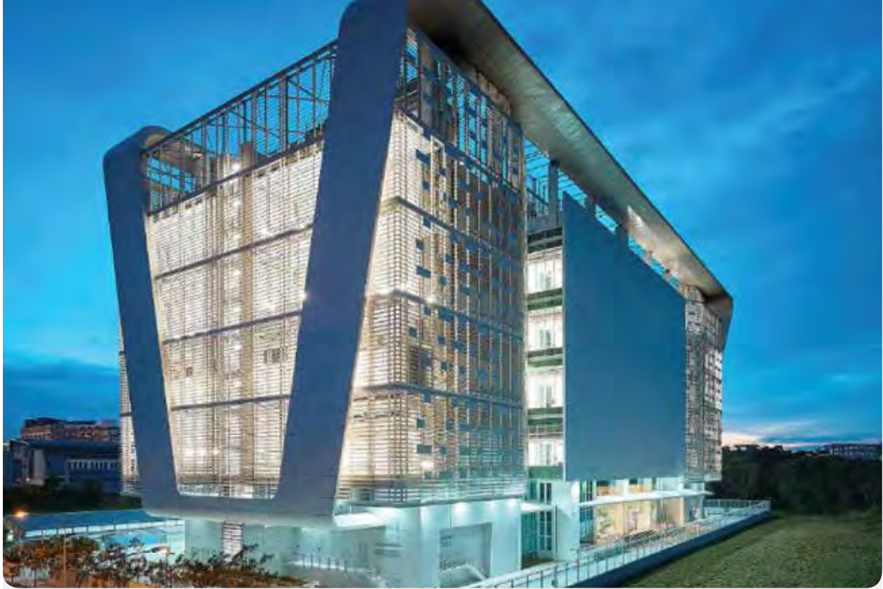
Telin-3 Data Center in Singapore.
