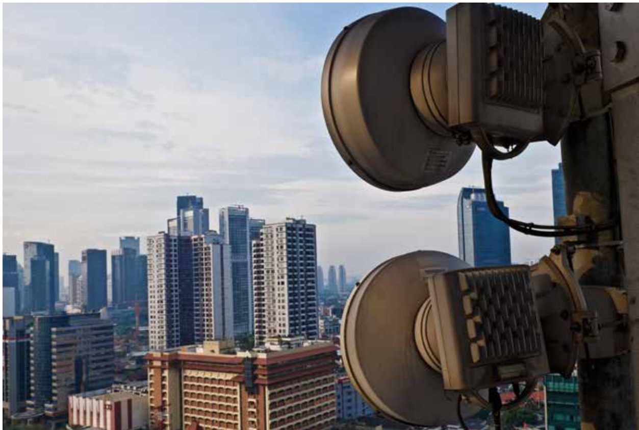
→ Outdoor Micro BTS is one solution to expand cellular coverage and increase the capacity in strategic location and central business district.
