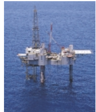
The completion phase of the well at Eugene Island Block 271/264 is shown below. Initial production began in August 2000, and the well is producing natural gas at a daily rate of 10 million cubic feet.
