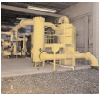
Horizon Power owns a 50% interest in this 5.6 megawatt power plant located near Lewiston, N.Y. Methane gas produced from an adjacent land-fill is gathered and treated before it is routed to fuel the seven engines which generate electricity to feed the power grid serving western New York.
