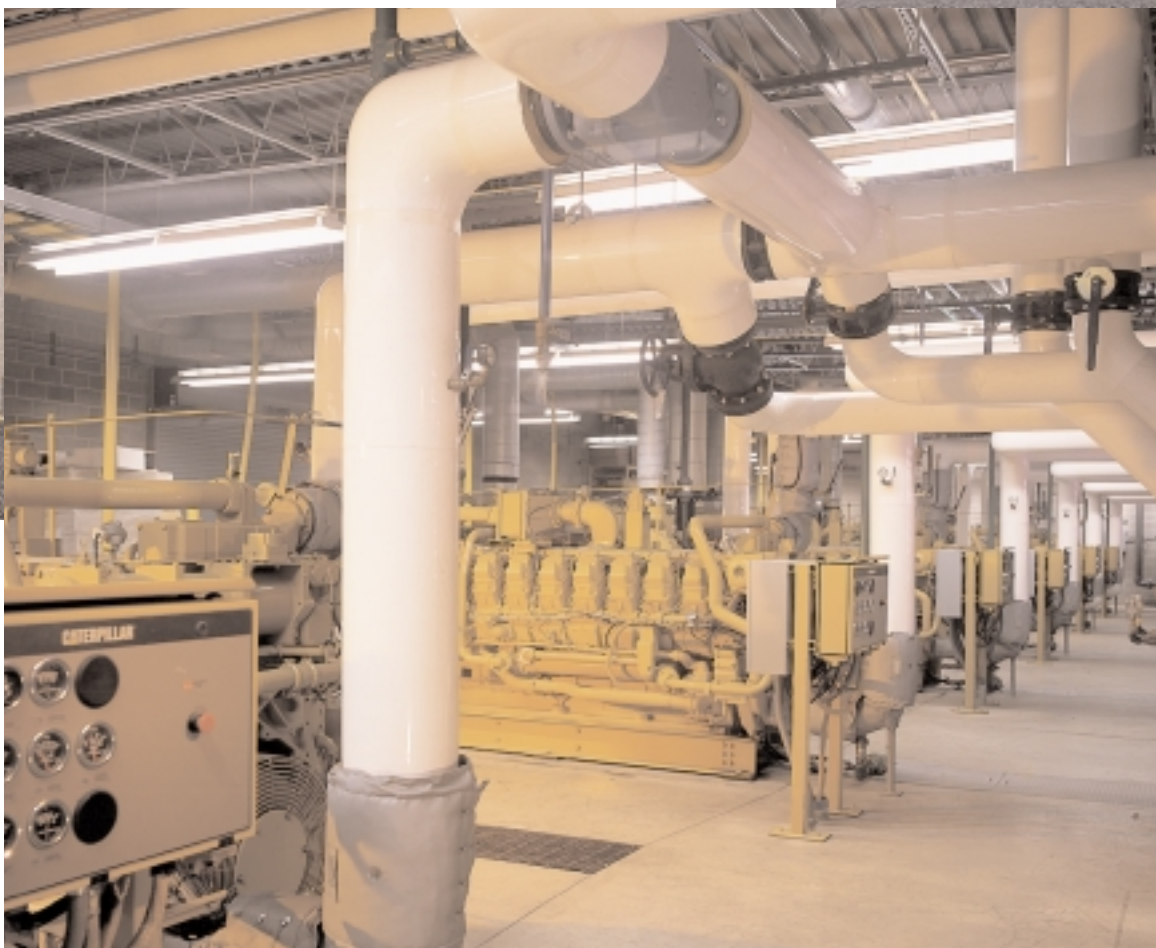
Horizon Power owns a 50% interest in this 5.6 megawatt power plant located near Lewiston, N.Y. Methane gas produced from an adjacent land-fill is gathered and treated before it is routed to fuel the seven engines which generate electricity to feed the power grid serving western New York.
