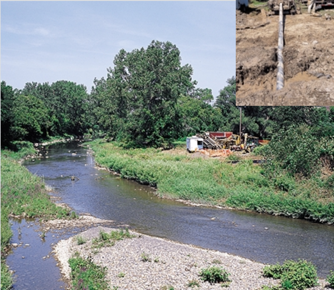
Approximately 4,000 feet of the Line K (1954 bare-steel) pipeline in West Seneca, N.Y. was replaced this summer with new 20-inch diameter coated steel pipe. This replacement is part of ongoing upgrades to the Pipeline and Storage transmission system. Horizontal directional equipment was used to bore a hole that was 940 feet long and 30 inches in diameter for the new pipeline to be installed underneath Cazenovia Creek and Ridge Road as shown here. This technique is environmentally friendly and the creek was not disturbed.
