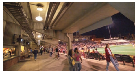
The Erie Seawolves (AA baseball) turned to National Fuel's Utility segment to help raise attendance at cold-weather games. The solution came in the form of "Heat Zones," radiant tube, high-intensity infrared heaters, that have helped increase attendance 17 percent in the season's two coldest months (April and May). As a result, two additional heaters will be installed in early 2006.
