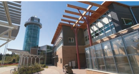
The Tom Ridge Environmental Center at Presque Isle, set to open to the public in 2006, recently earned the prestigious Leadership in Energy & Environmental Design (LEED) accreditation from the U.S. Green Building Council, thanks in part to the high-efficiency natural gas boiler system chosen for this state-of-the-art, 60,000 square-foot facility. It is the first structure in Erie, Pa., to receive LEED certification.
