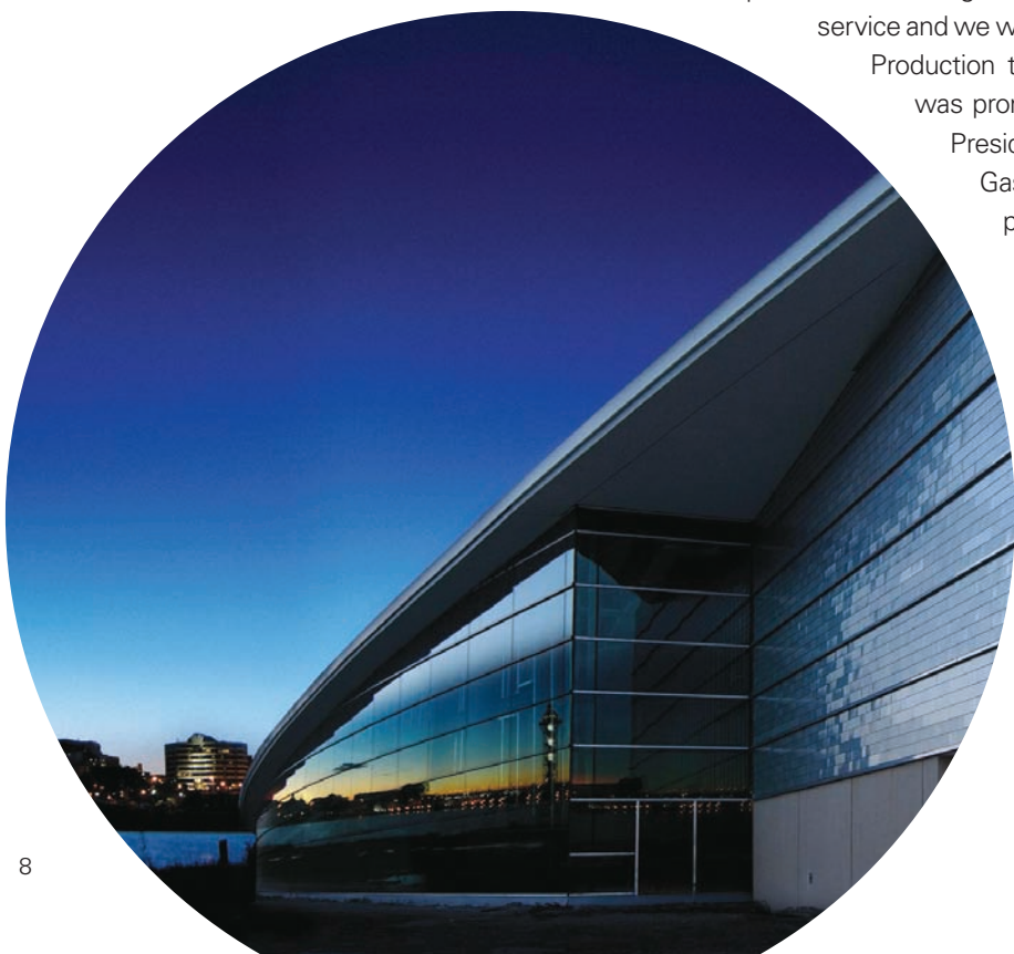
The new Bayfront Convention Center, located on Lake Erie's Presque Isle Bay in Erie, Pennsylvania, opened in the summer of 2007. This $44 million facility is the largest development in the City of Erie's history and is expected to increase the Utility segment's throughput by approximately 13,400 Mcf per year.
