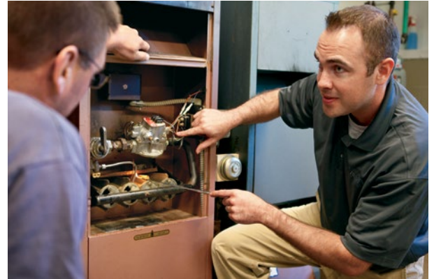
▲ Utility employee Todd Woods demonstrates how to re-light natural gas appliances in the company's new state-of-the-art training facility.
