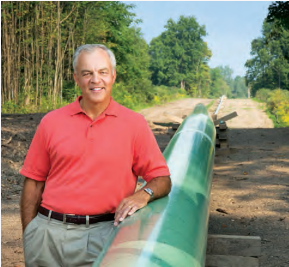
Ron Tanski, President & CEO, is pictured along Supply Corporation's NM-44 line in Elma, N.Y., where four miles of transmission pipeline were replaced in 2015 as part of the Company's ongoing modernization and safety program.
