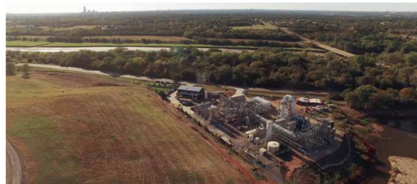
The ENVIA plant and the East Oak landfill site in the foreground with downtown Oklahoma City just visible on the skyline (left). The plant is co-fed by landfill gas produced at the adjacent landfill site and pipeline natural gas.
