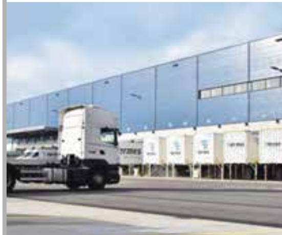
Hermes facility, Hamburg • Germany
