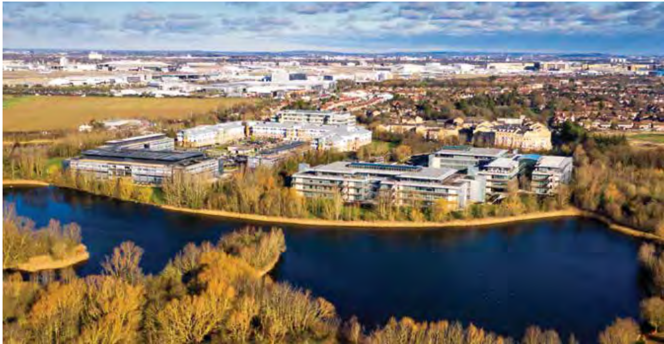
▲ Lakeshore, Bedfont Lakes Business Park, Heathrow • United Kingdom
