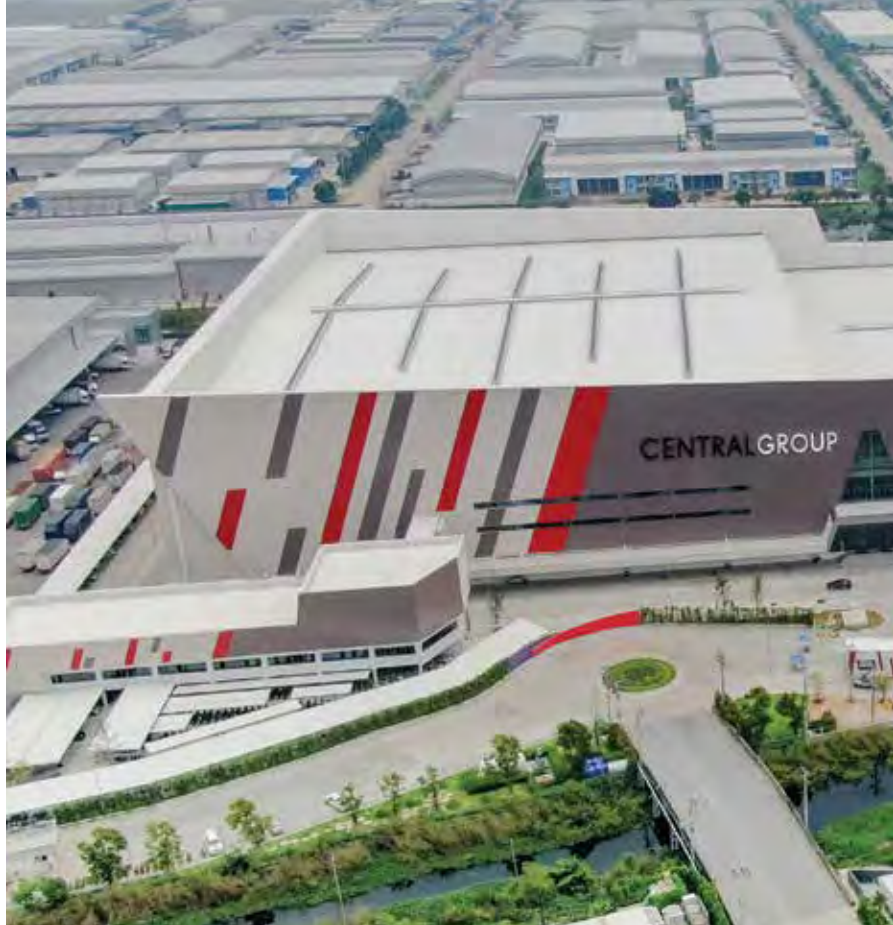
▲ Build-to-suit Central Retail facility, Bangkok • Thailand
