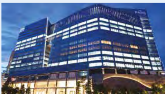
▲ The PARQ in Bangkok • Thailand. Tenants can monitor indoor air quality and control SMART lighting systems through a mobile app.
