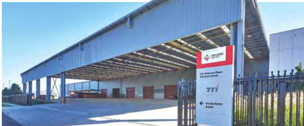
▲ TTI, Eastern Creek Business Park, New South Wales • Australia
