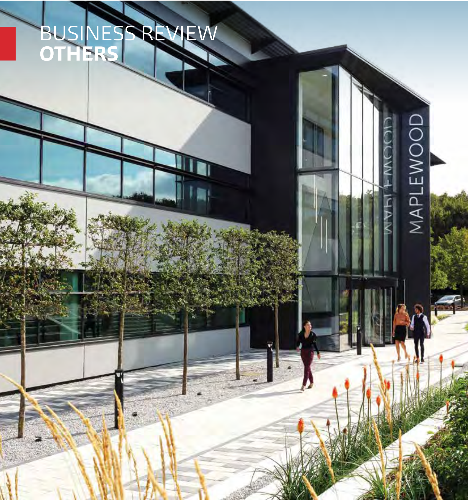
▲ Maplewood at Chineham Business Park, Basingstoke • United Kingdom
