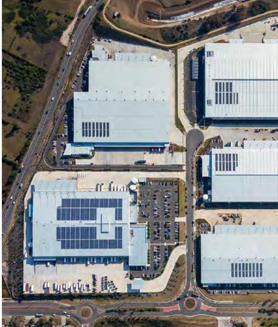
▲ The Horsley Park Estate, New South Wales • Australia
