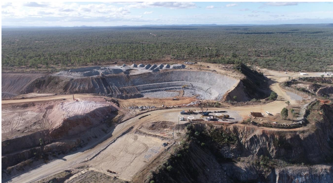
Pictured above: K2H Wises Dam – Placement of embankment fill
