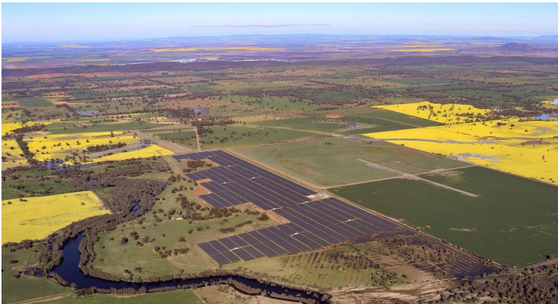
Above: 50MW Jemalong Solar Farm, Central NSW
