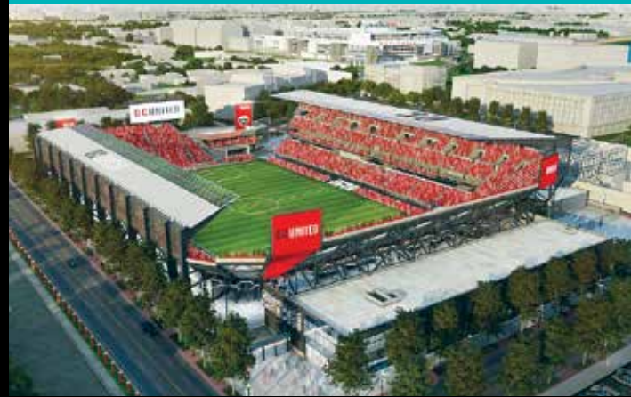
Project: DC United Soccer Stadium Customer: Turner Construction Company Location: Washington, DC
