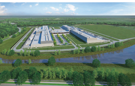
Customer: Turner Construction Project: Turnstile (Confidential) Location: New Albany, OH
