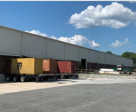
COSENTINO DISTRIBUTION CENTER Rincon, GA (Savannah MSA) Industrial
