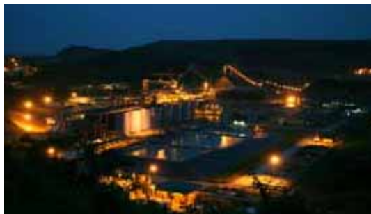
CIL plant at night.
