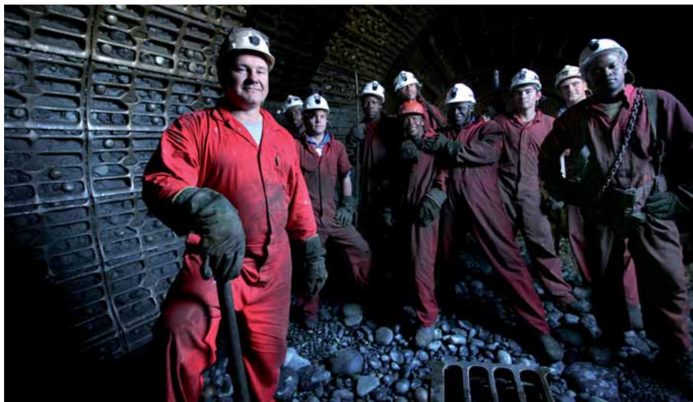
Crew replacing liners inside mill at Beatrix
