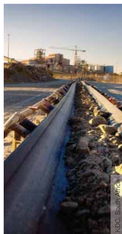
Welding at Agnew, Australia
