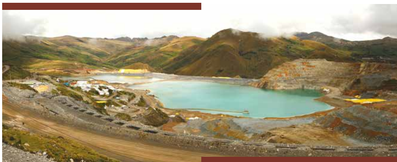
Tailings facility at Cerro Corona in Peru
