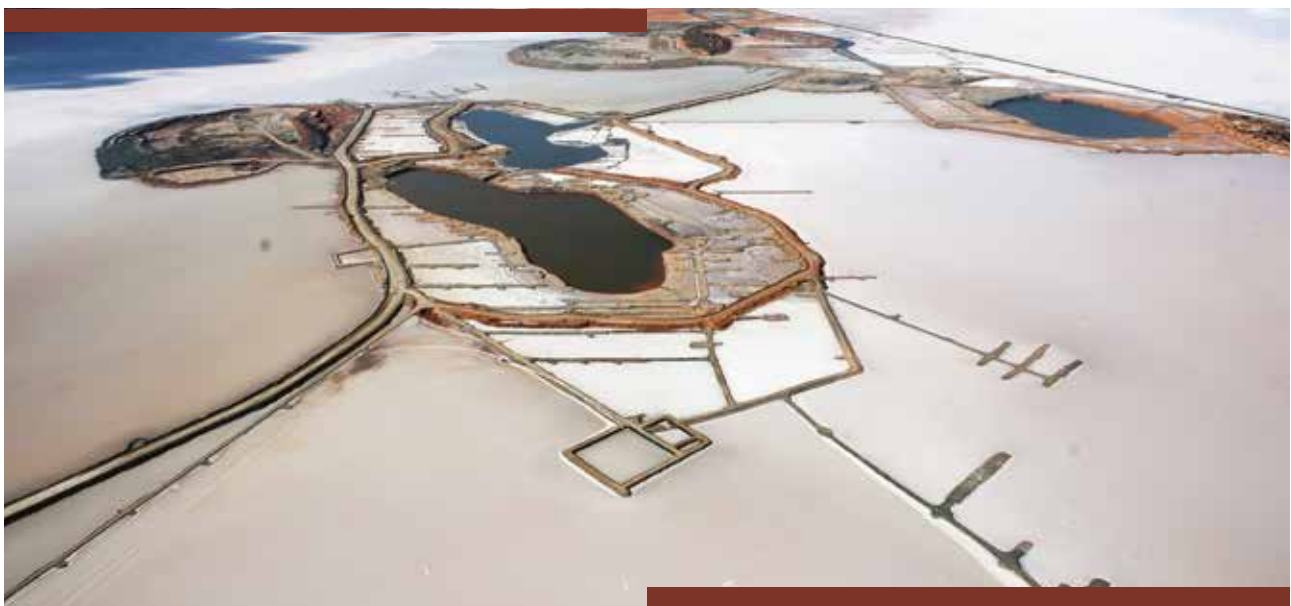
Causeways onto Lake Lefroy, at the St Ives gold mine
