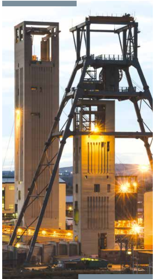
Twin shafts at the South Deep mine in South Africa
