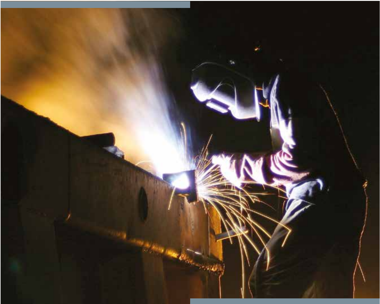
Boilermaker at work at Tarkwa mine in Ghana
