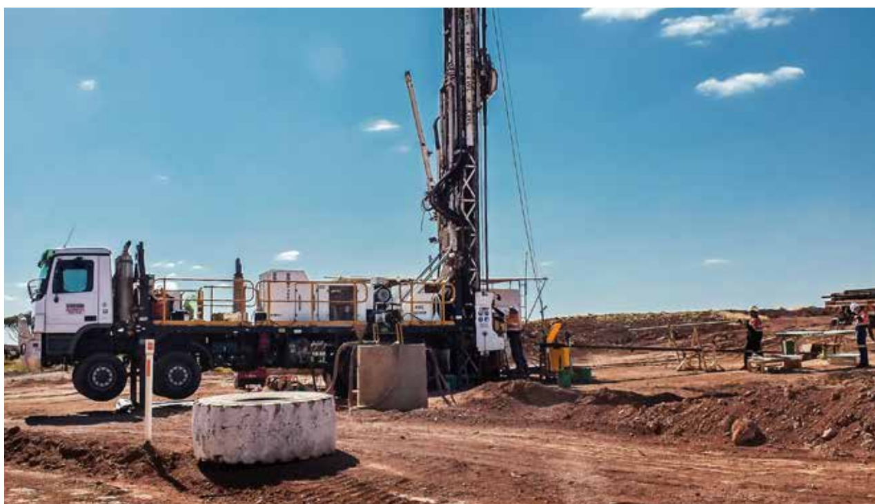
▶ Borehole drilling at our Australian operation
