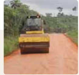
Road repair near Tarkwa
