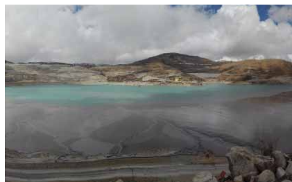
Tailings storage facility at Cerro Corona, Peru
