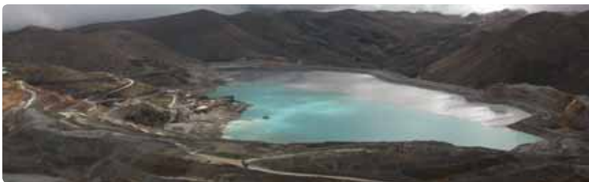
Cerro Corona tailings storage facility
