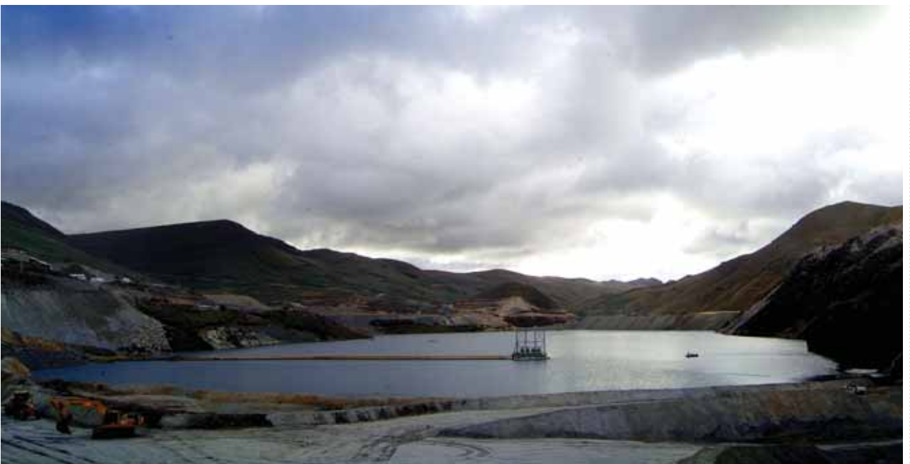
Tailings Storage Facility at Cerro Corona, Peru
