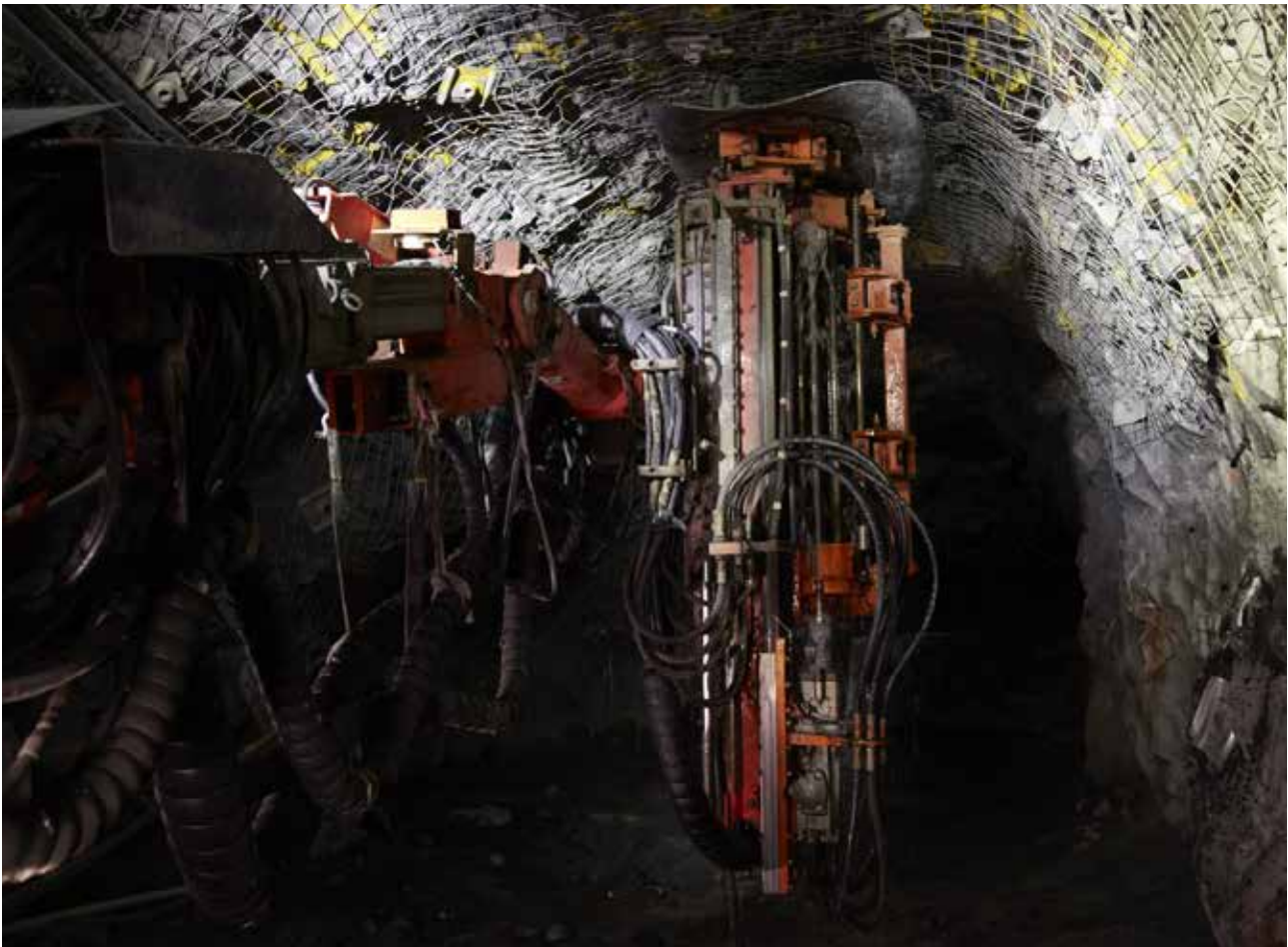
Pinning wiremesh to the hanging wall at the Agnew mine
