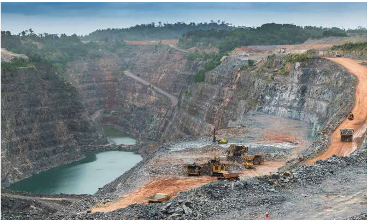
Work at the Damang pit cutback project
