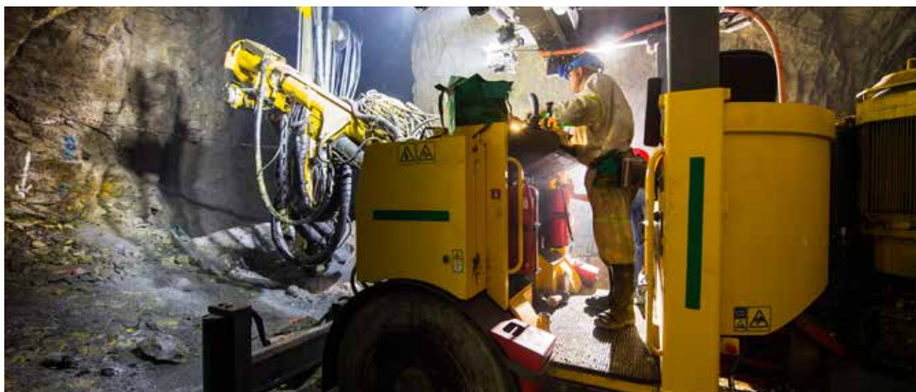
Drilling and installing support at South Deep
