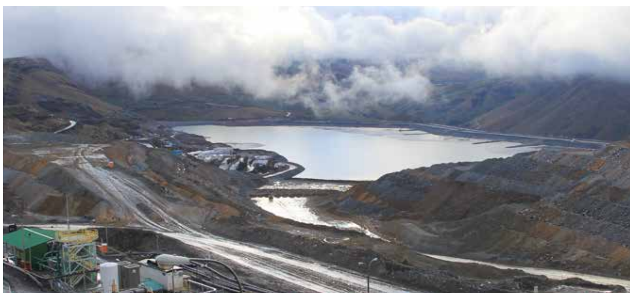
Tailings storage facility at Cerro Corona
