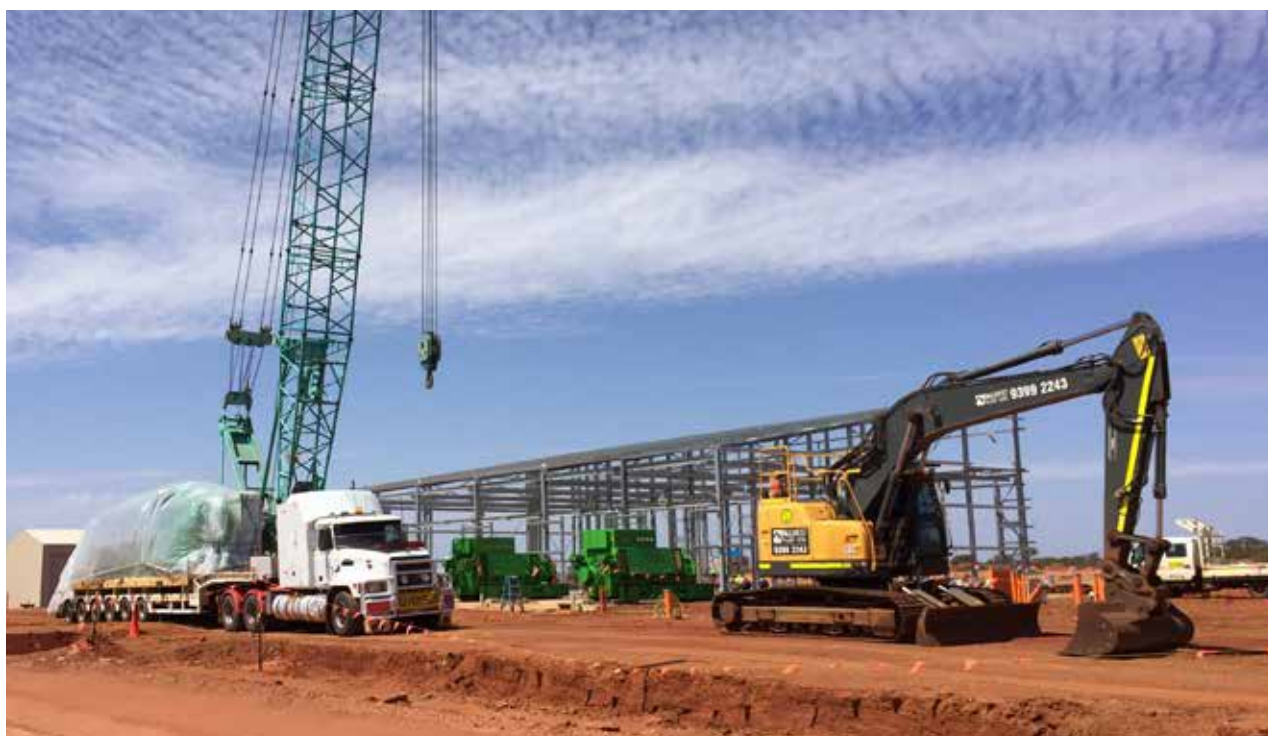
Construction and civil works at the Gruyere project in Western Australia
