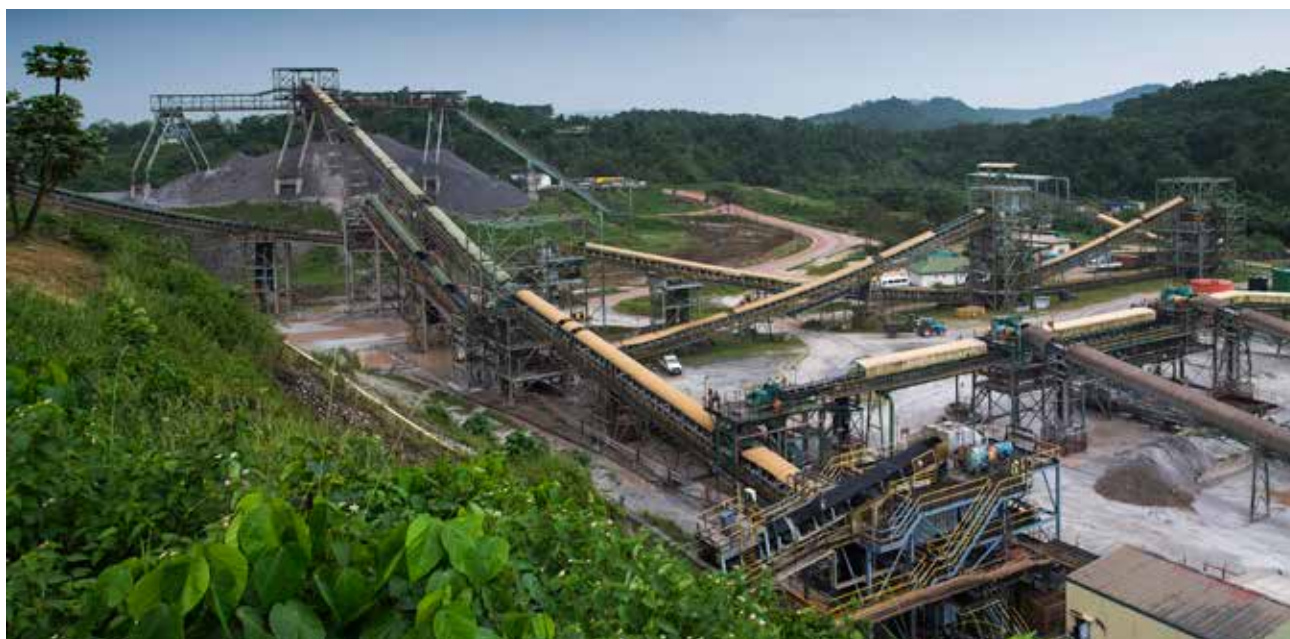
Conveyor belts feeding the crushing and metallurgical plant at Tarkwa
