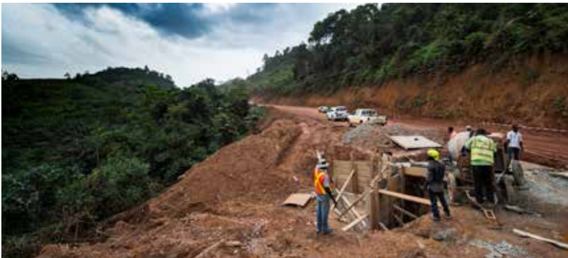
Rehabilitation of the road between Tarkwa and Damang
