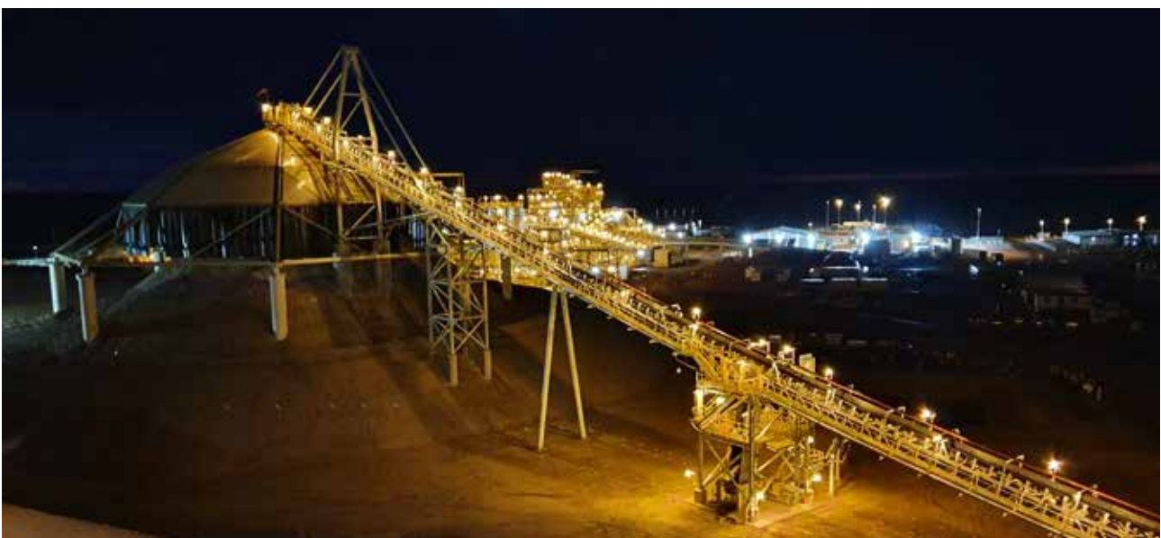
Ore conveyor belt at our Gruyere mine in Australia
