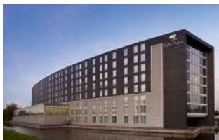
Park Plaza Amsterdam Airport Close proximity to Amsterdam Schiphol Airport 342 rooms
