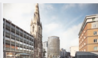
LONDON PIPELINE, UK
