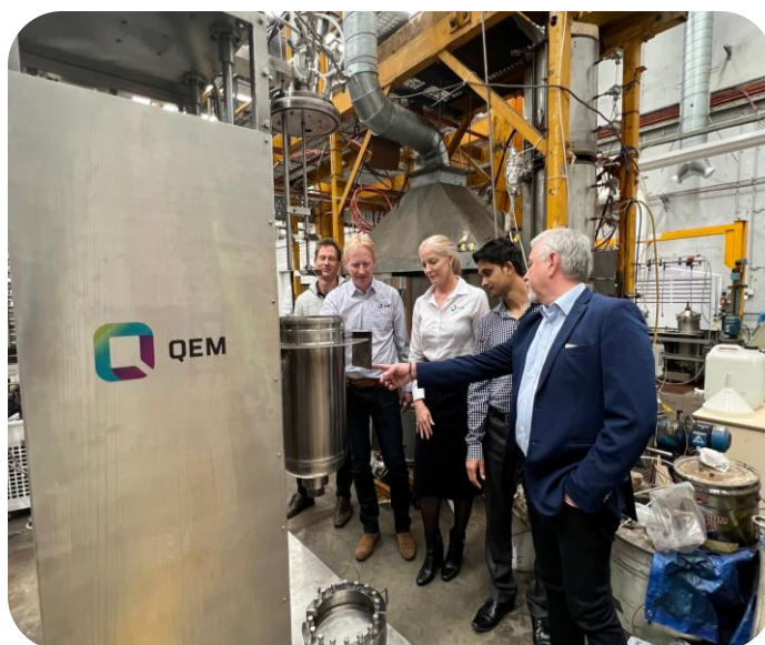
The installation and commissioning of the bench scale pilot plant at HRL's Melbourne headquarters during FY22.
