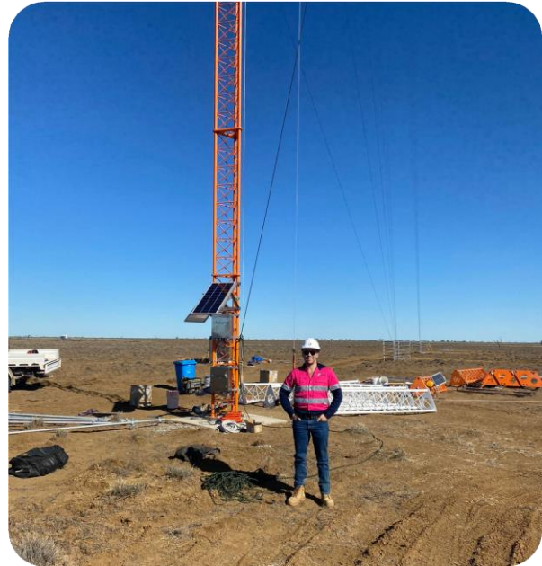
Images: SODAR and Solar equipment installed on site at Julia Creek; 160m Met Mast commissioned on-site July 2022
