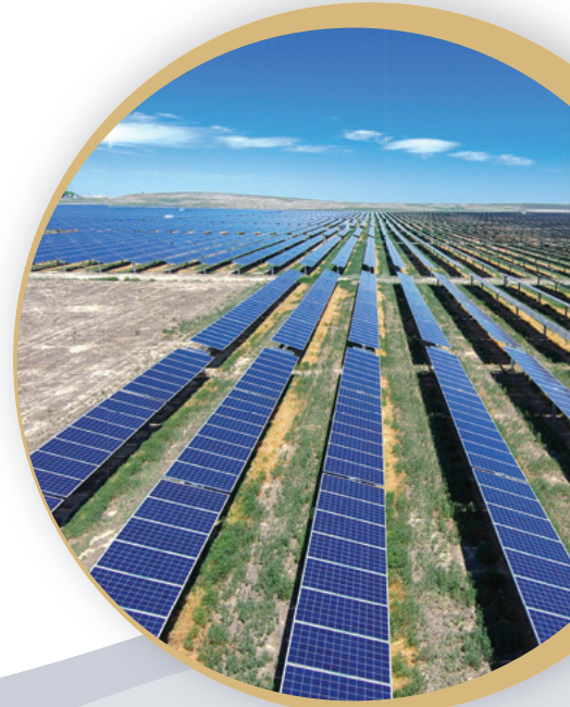
C.J. Strike Solar Facility
