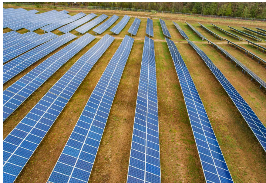
Oak solar farm in New Jersey, US is comprised of 53,200 fixed solar panels and has a capacity of 10MW.
