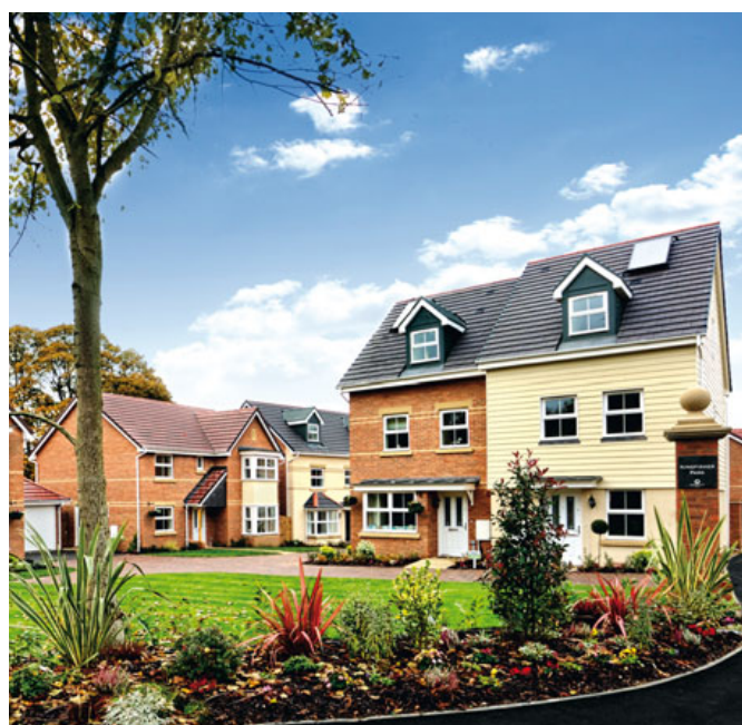
A brand new community of houses and apartments at Kingfisher Park in Buntingford, Hertfordshire.
