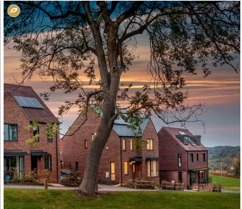
The David Wilson Homes and Barratt Homes award winning hillside development in Coulsdon, Surrey. The site showcases 659 quality homes with far reaching views and Built for Life accreditation.
