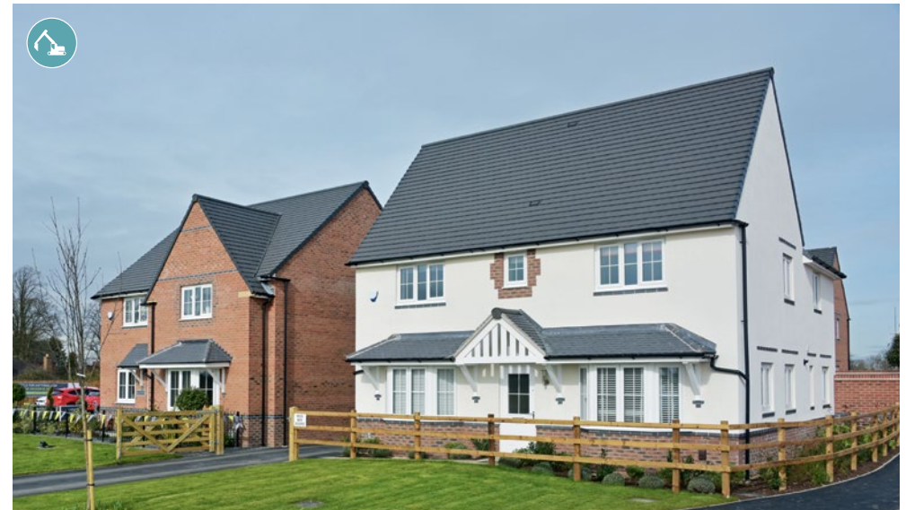
Large format block was successfully trialled in the construction of 34 homes at The Wickets development in Bottesford, near Nottingham.
