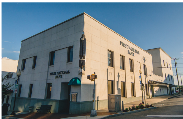
Altavista Main Office – Corporate Headquarters
