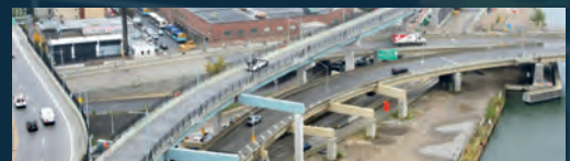
RFK Bridge Connector Ramp eliminated 2,500 tons of CO 2 e per year.
