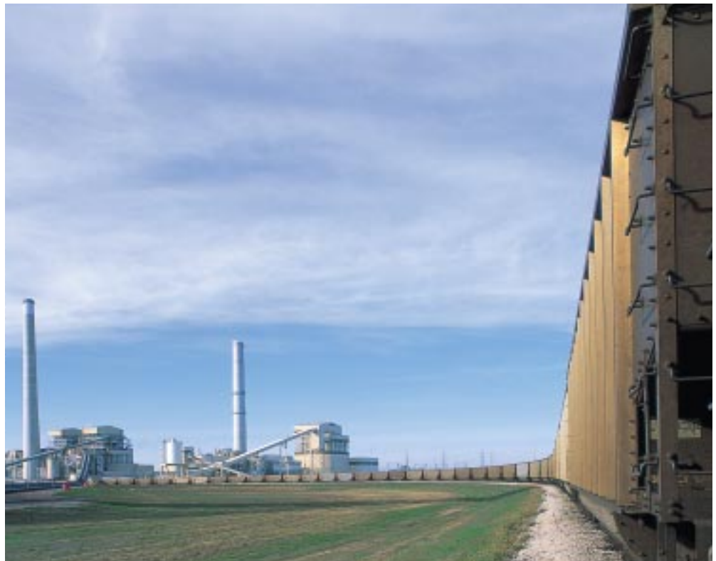
Above: Unloading Powder River Basin coal at San Antonio City Public Service, a customer of Rail Link.
