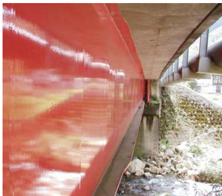
A bridge beam (in its 21 st year) with LUMIFLON coating
