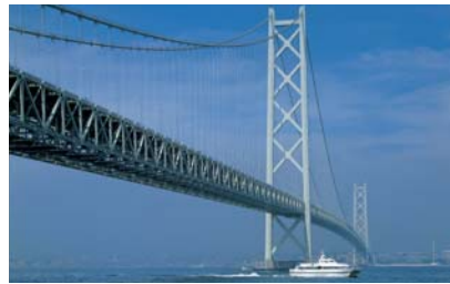
The Akashi Kaikyo Bridge, treated with highly weather-resistant Lumiflon™ fluoropolymer coating
