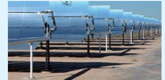
Glass mirrors for solar thermal generation
