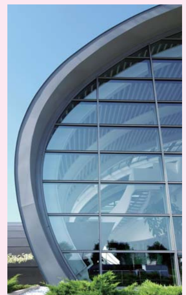
AGC's Low-E glass is used in various locations worldwide (Photo: Padova, Italy) ©AGC Glass Europe
