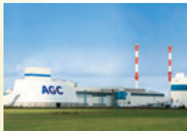
Klin Plant, located approximately 80 km northwest of Moscow
