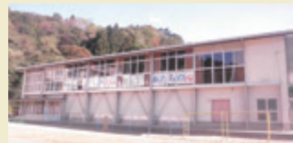
The gymnasium of Hashiura Municipal Elementary School in Ishinomaki City, a laminated glass for earthquake/typhoon resistance recipient
