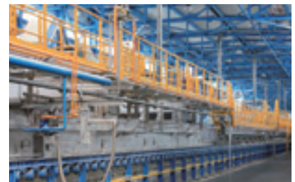
One of the largest glass manufacturing facilities in the world, in the Klin Plant
