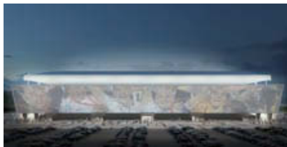
The east façade of the Arena Corinthians stadium utilizes Planibel Clearvision, a high-transmission glass
